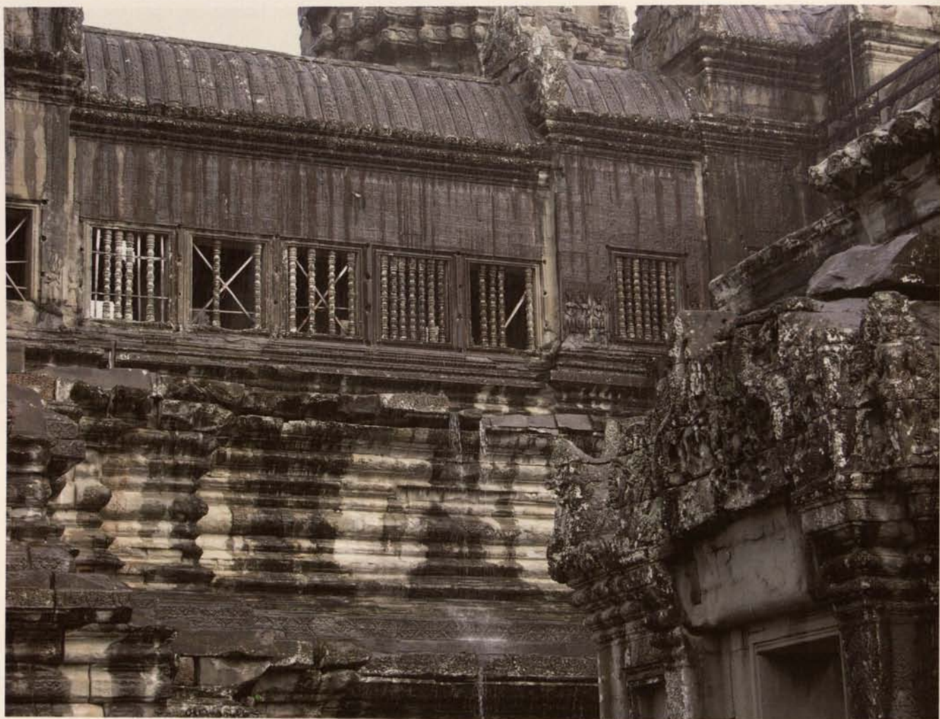
Fig. 9. Angkor Vat, temple: The removal of the natural biofilm led to the overgrowth of blackening microorganisms with additional thermal-hygric stresses to the sensible claycontaining sandstone resulting in a severe detachment of rock shales from Apsara carvings.
