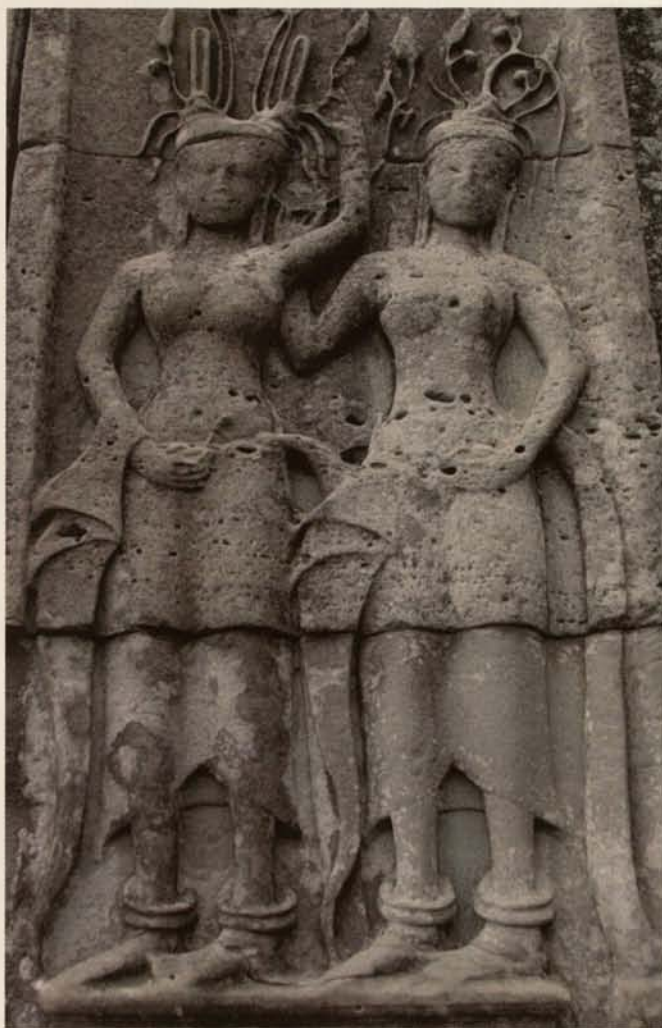
Fig. 11b. Angkor Vat, northern bibliotheca, detail: Successful application and longterm efficient protection of a specific designed biocidal formulation (four years after treatment).
